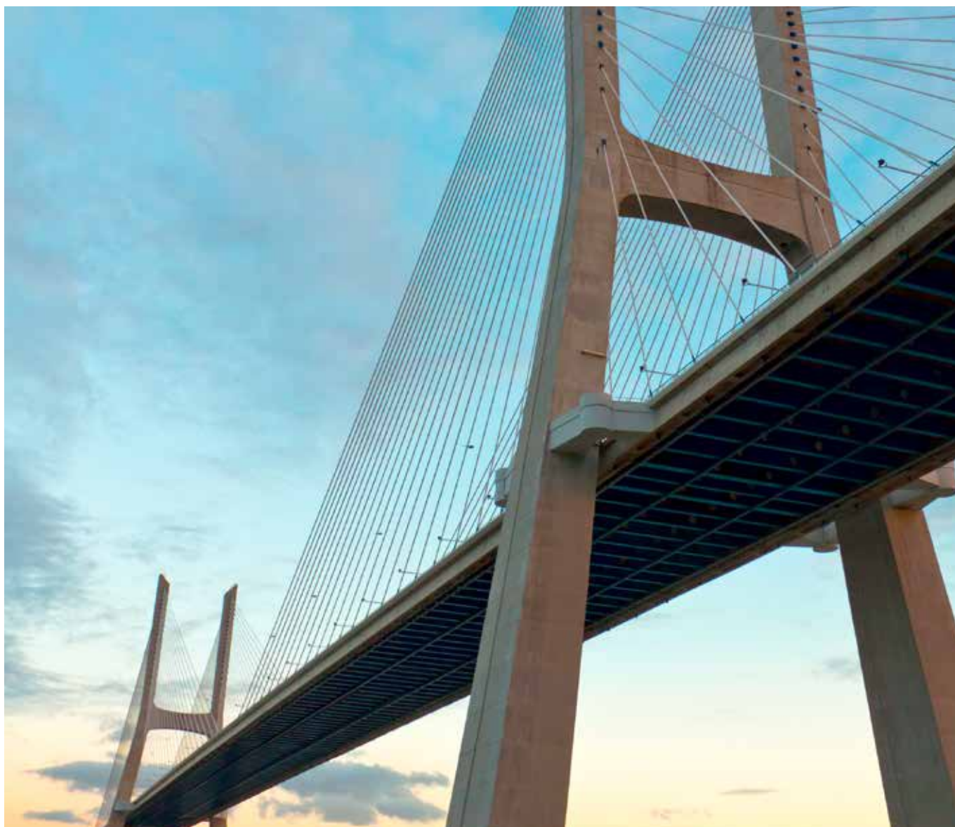
Vasco da Gama Bridge, Lisbon, Portugal
